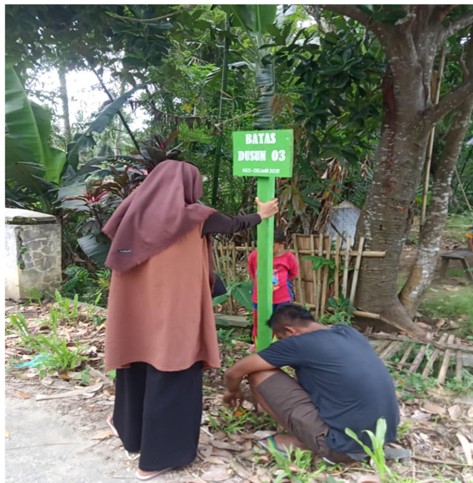
Figure 5. Laying Hamlet Boundary Barrier
